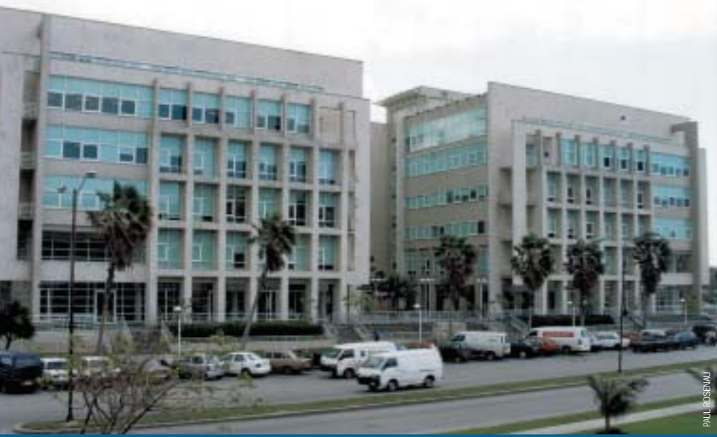
Havana's largest real estate joint venture project with over 1.8 million square feet of commercial space, the Miramar Trade Center has been called by local developers "Havana's Canary Wharf."
